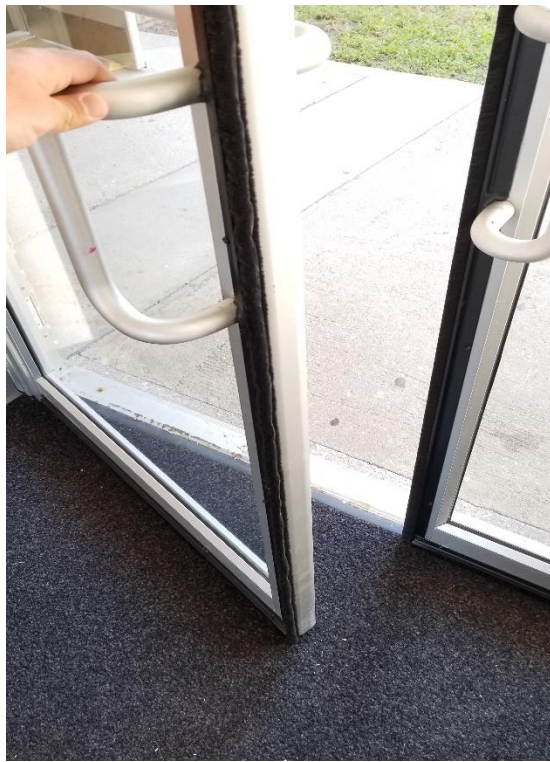
New weather stripping and door sweeps installed at Thorp Hall.
