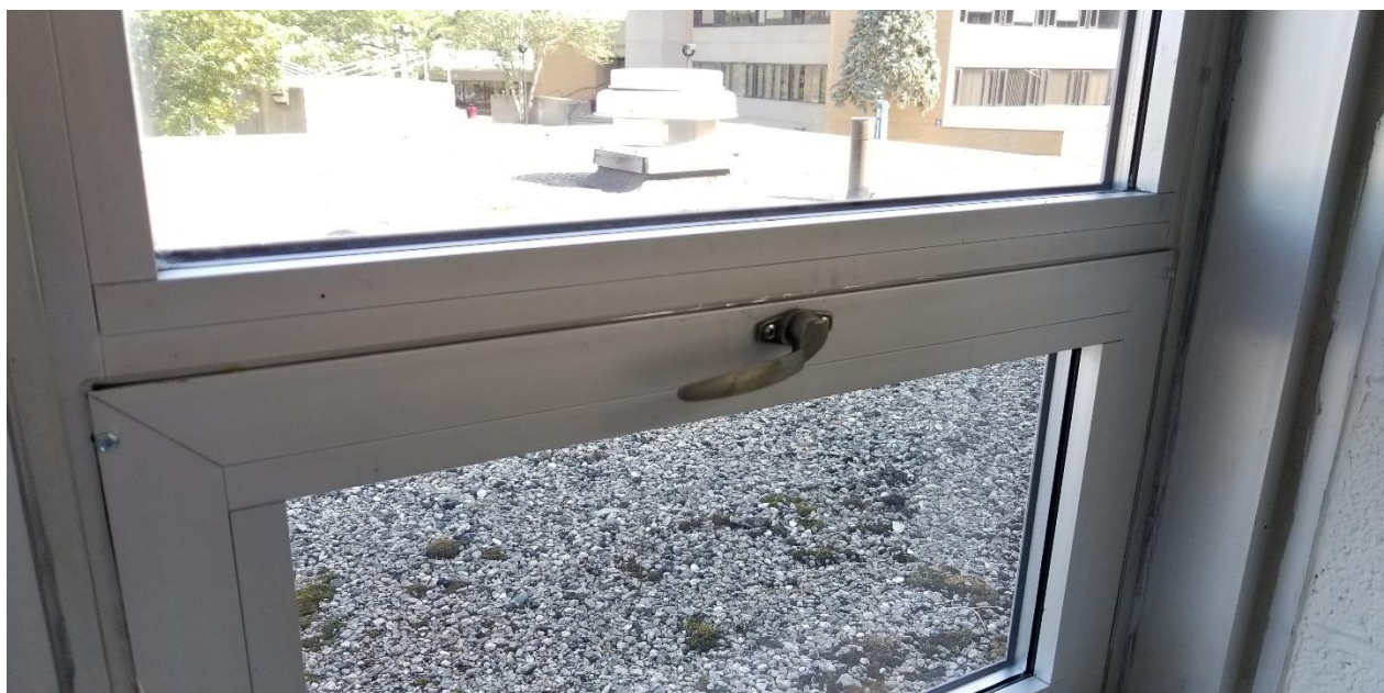
Common area windows caulked and sealed in Thorp Hall.
