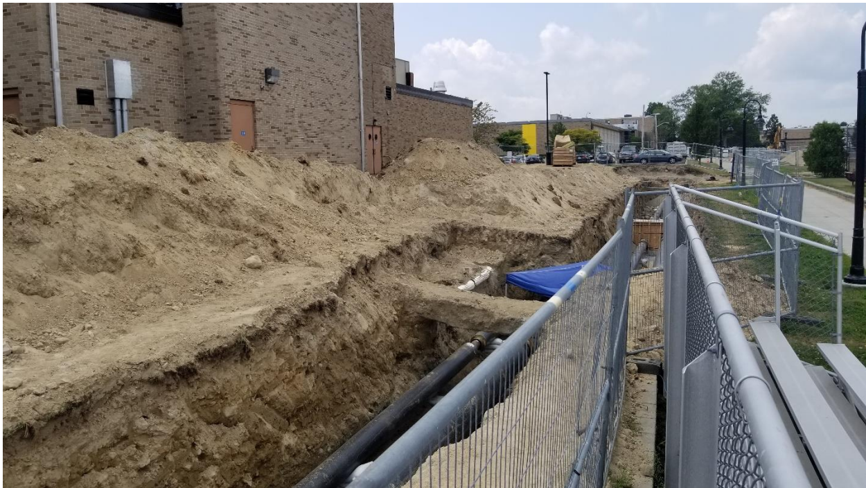
New high-pressure steam line connecting into Whipple Hall.
