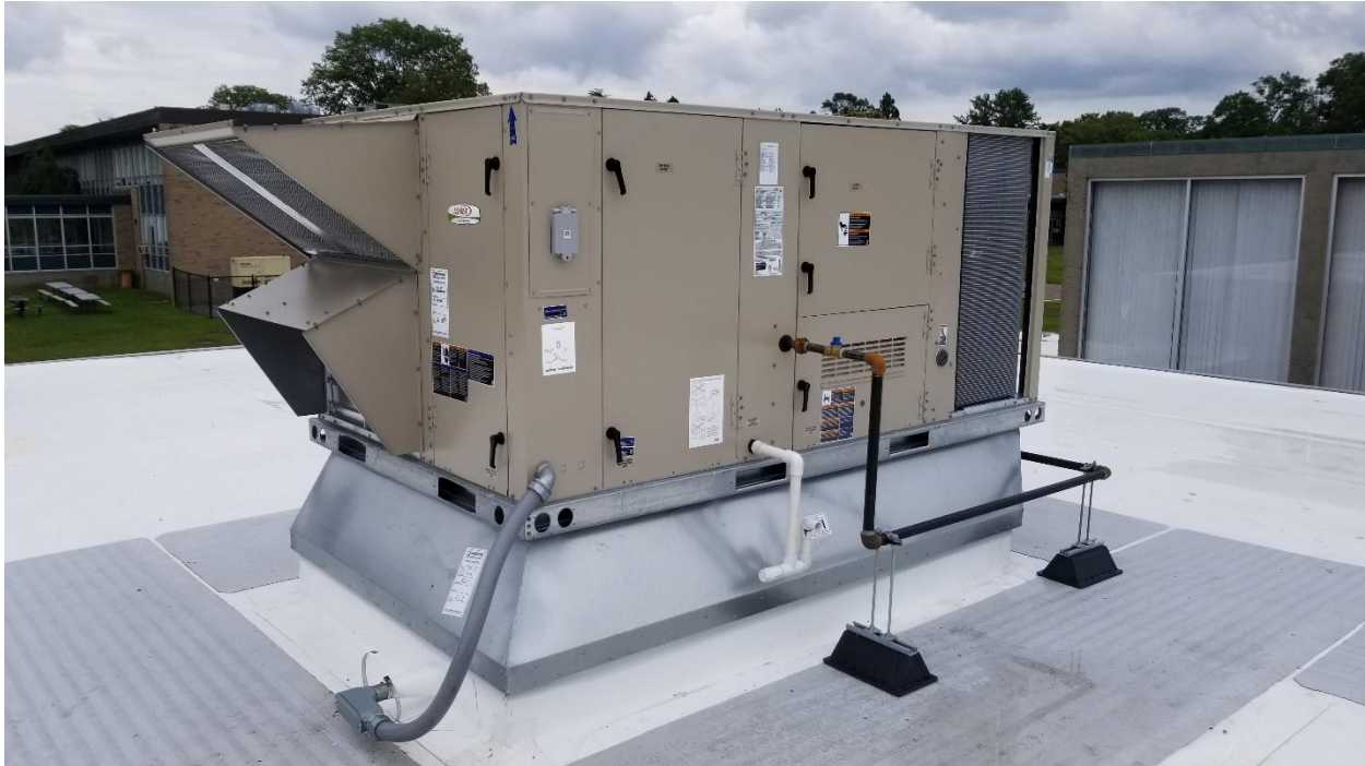
One of three new roof top units installed at Donovan Dining Hall.
