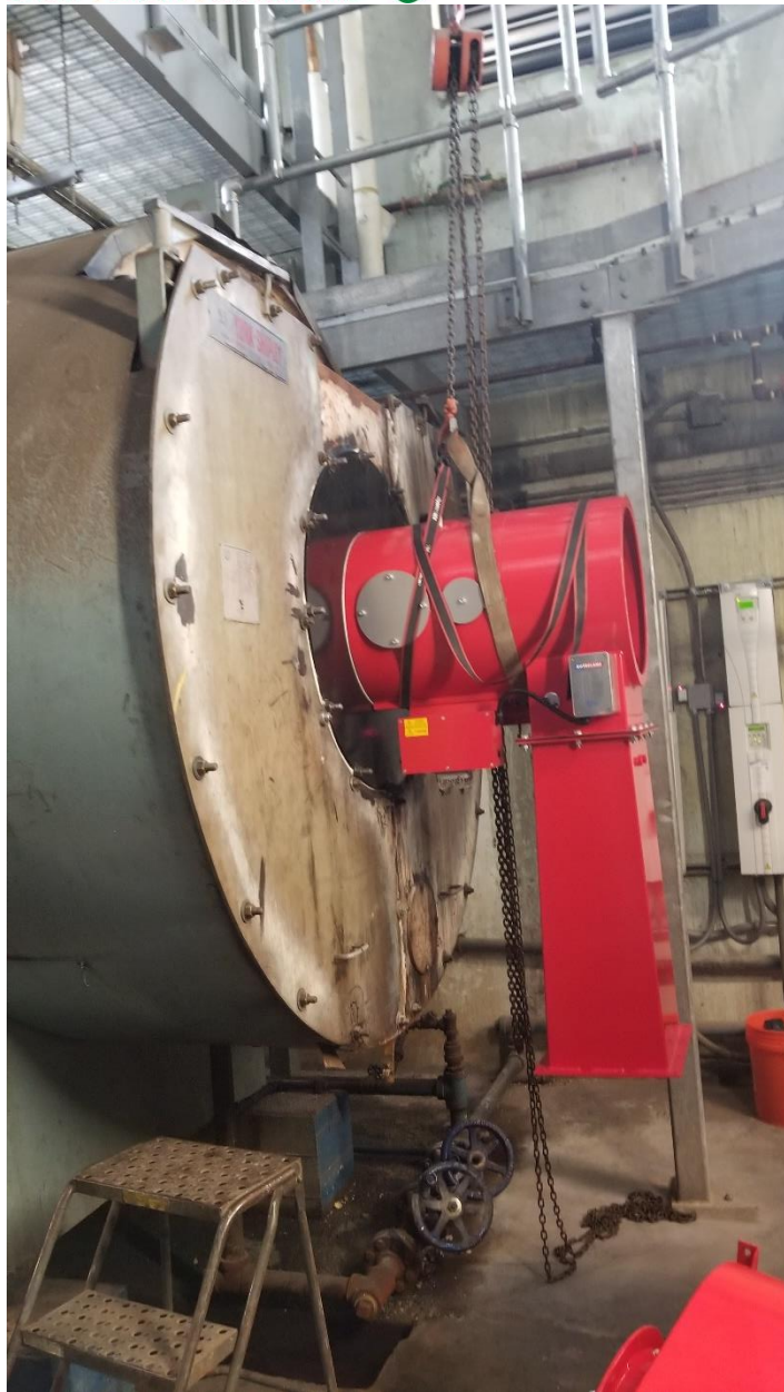
New high efficiency burner being installed in the central heating plant.
